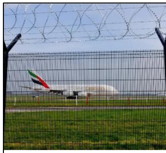
Figure 5.18: Illustration of welded steel mesh used for fencing (railway)
