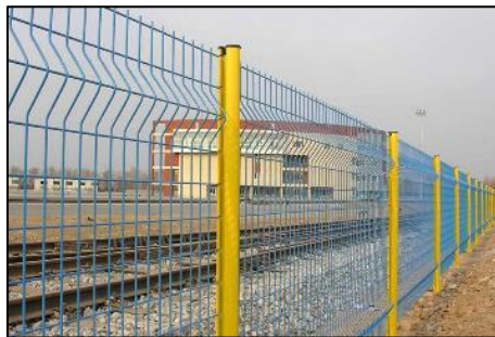
Figure 5.18: Illustration of welded steel mesh used for fencing (railway)
